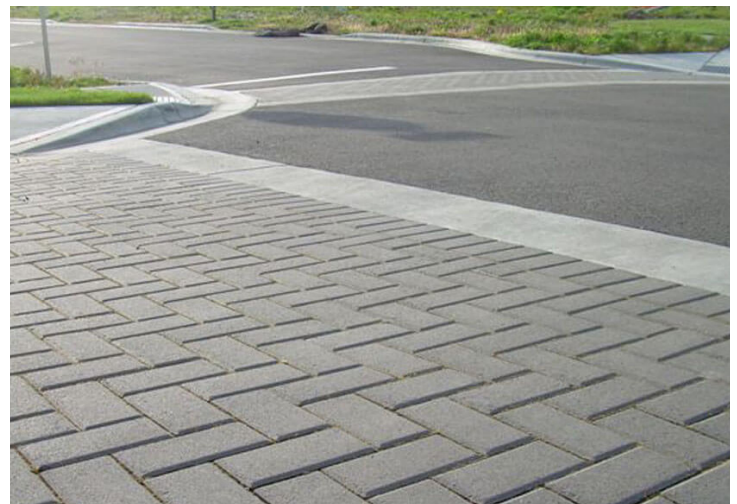
Figure 6.2: Paver crosswalk with concrete band and asphalt road.
