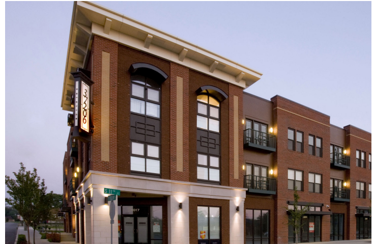
Figure 5.3: Example of a projecting sign on a signature building corner.
