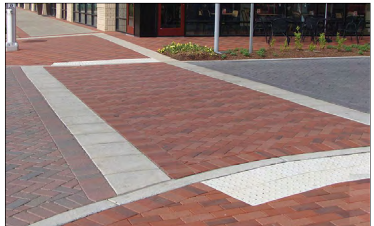
Figure 6.3: Crosswalk materials shall be pavers with concrete banding or concrete pavement on either side.
