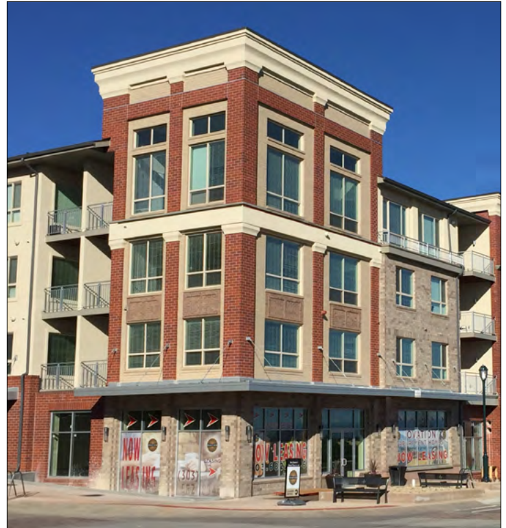
Figure 2.4: Permitted masonry products include brick and stone, including the synthetic versions of these products.
